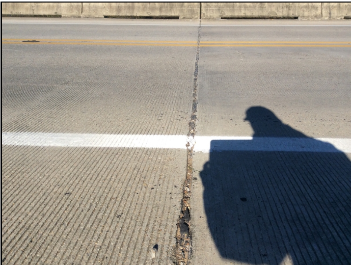
JOINTS NEED TO BE CLEANED AND SEALED ALL SPANS
